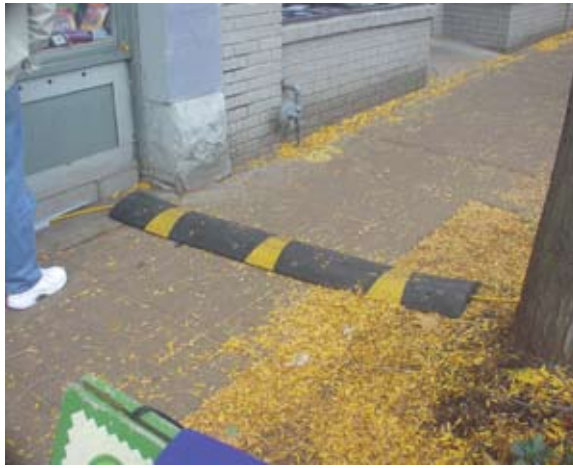
If you have to run an electrical cord across a walkway, cover it with a cord cover like this one, seen at a farmers market in Seattle. Photo by Zachary Lyons.
